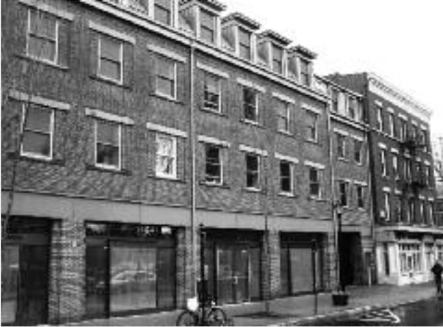
The window openings, roof line, and materials of this new mixed-use building in New Haven, Conn., (left) are compatible with the historic buildings further down the block.
